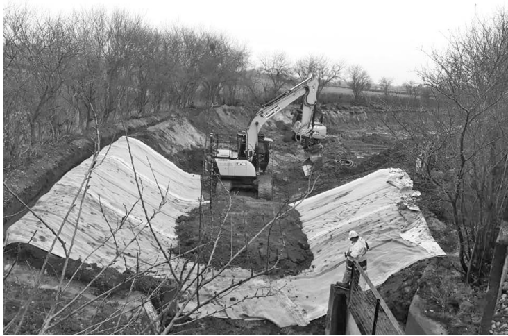
Laying the lining of the canal
